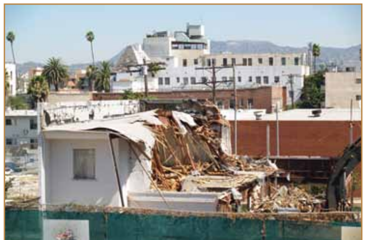
Demolition of 6th and Harvard property begins
