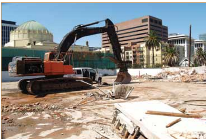
Leveling of the new property
